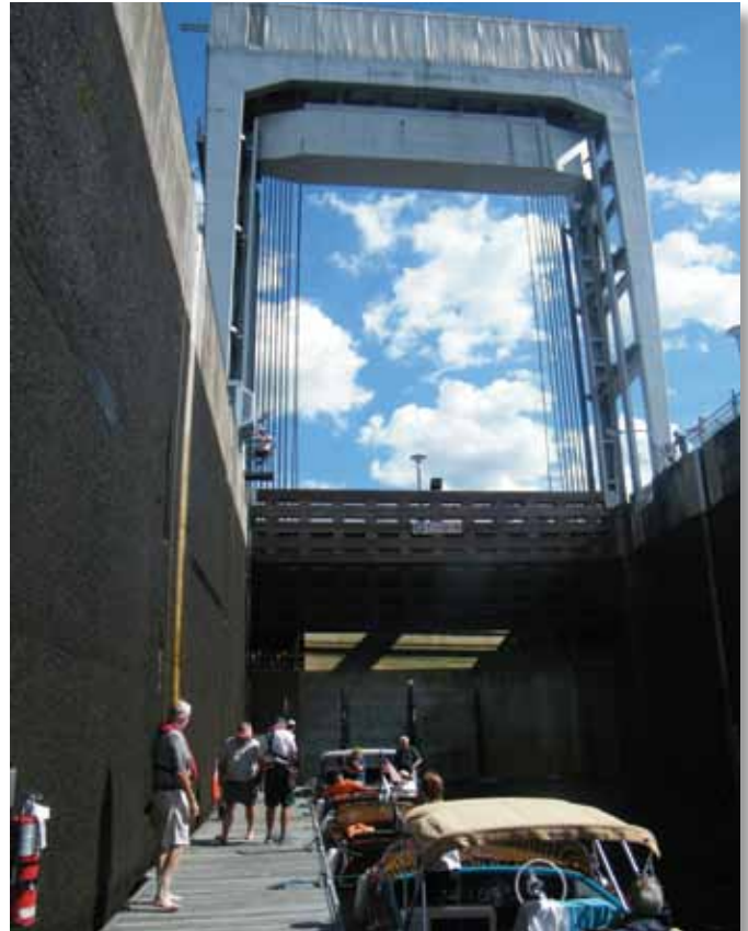
The Carillon Lock with its unique guillotine closing system.
